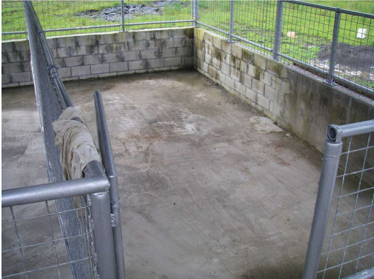
Figure 2 – Individual Pen before Addition of Litter – 12' Wide x 24' Long x 3' Deep
