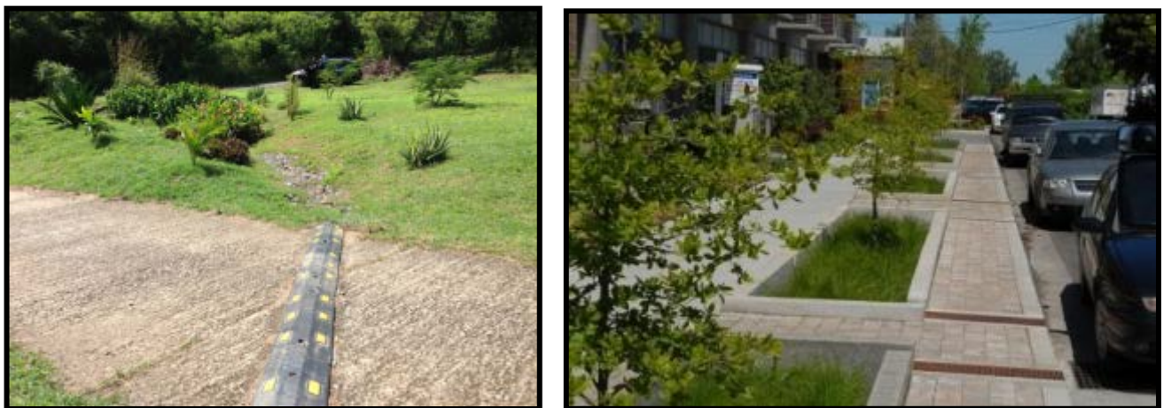
Figure 12. Rain garden from St. Croix and streetscape biofilters from Santa Monica, CA
