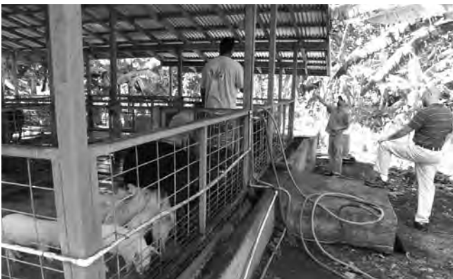
Wash down piggery system with waste washed into the trough. Solids are filtered off and composted; liquids are treated in a septic system and discharged to a drain field.
