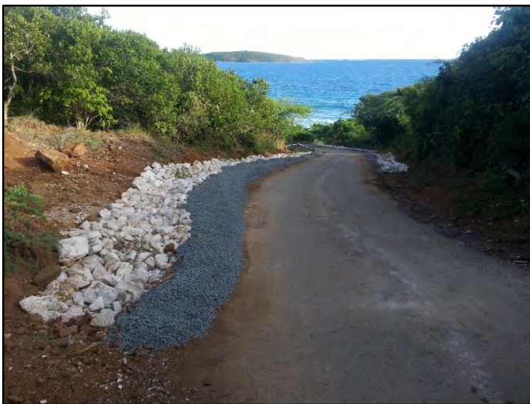
Figure 15. Riprap and Vetiver Swale.
