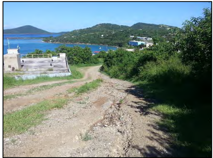
Figure 27. Dirt access road to the water tank prior to stabilization.
