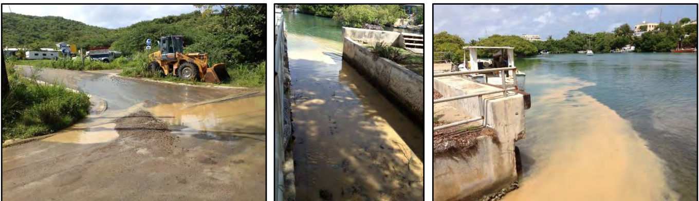
Figure 28. Water tank overflow prior to stabilization.
