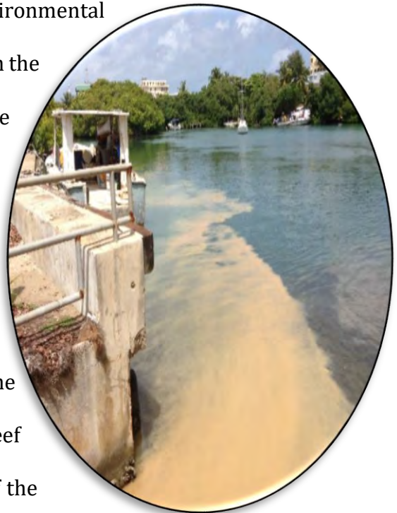
Figure 3 (Top). Runoff with fine sediments and beach erosion problems at Zoní Beach prior stabilization. Picture from the UPRM Sea Grant Program Marejada Magazine. Figure 4 (Bottom). Sediment plume out to the Lobina Channel from the town site prior stabilization.
