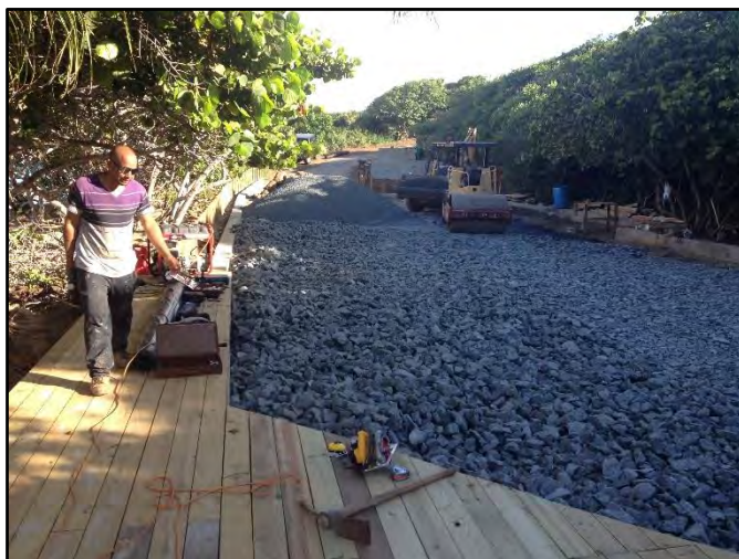
Figure 22. Parking filtration system construction.
