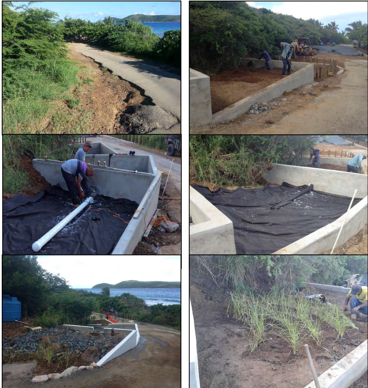
Figure 18. Construction of Filtration System.
