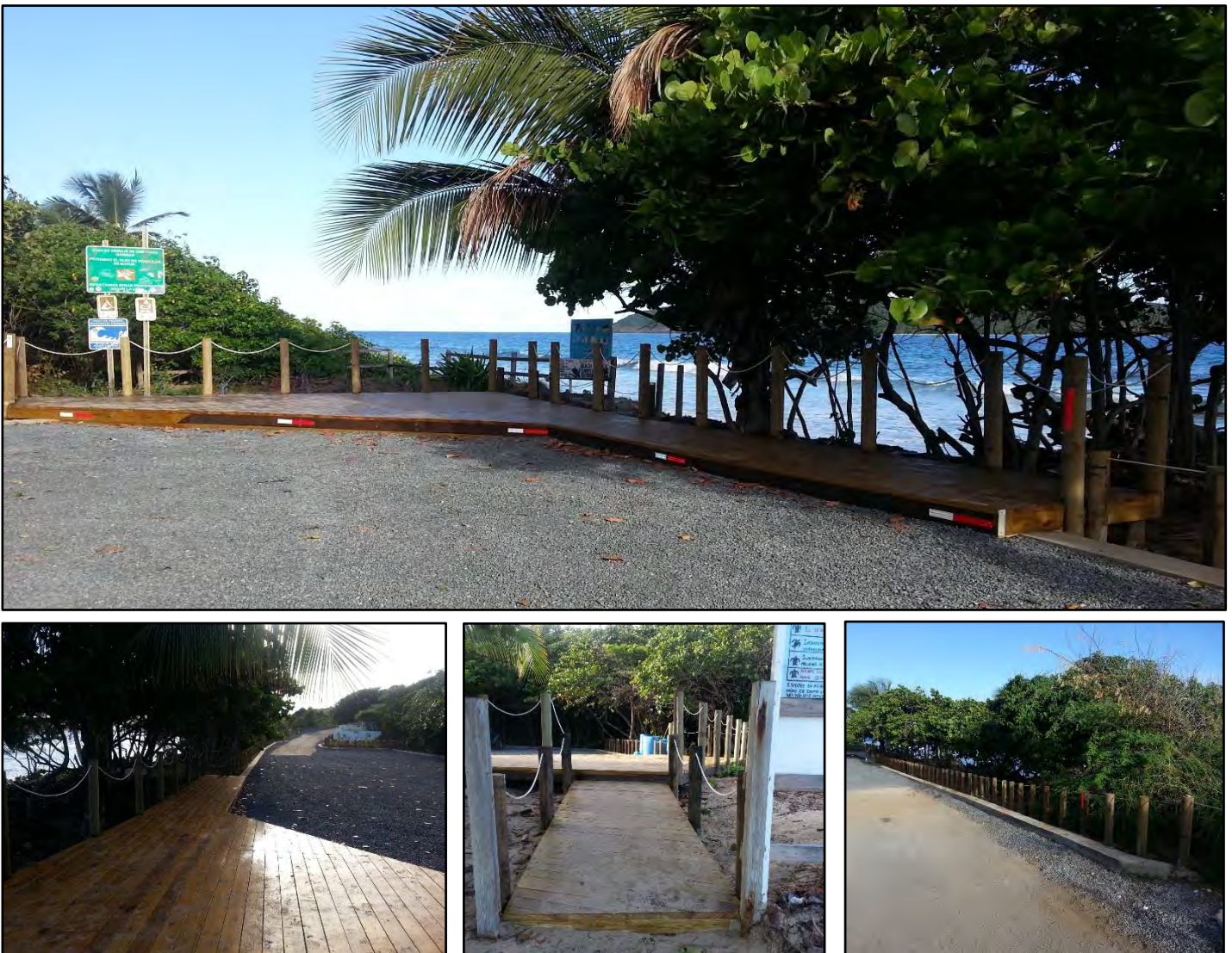
Figure 25. Elevated boardwalk and access delimitation.
