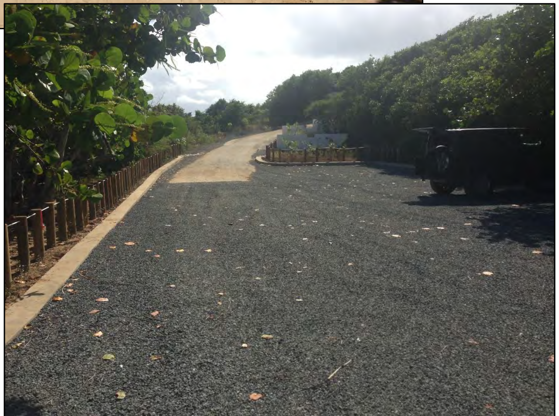
Figure 24. Parking area pre (top) and post (bottom) system construction.
