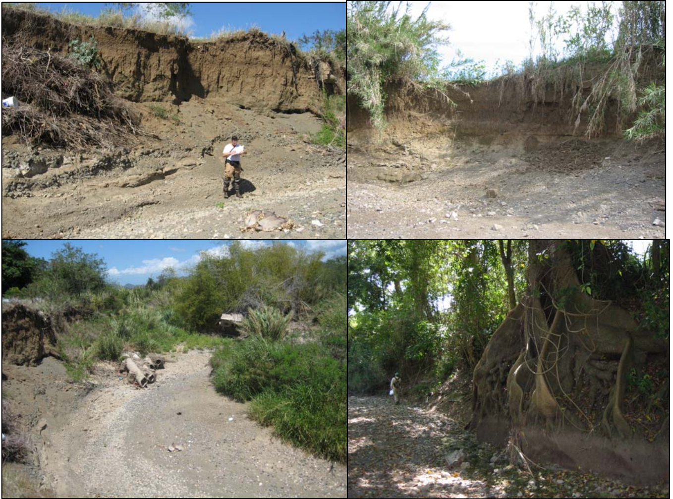
Figure 5. Channel erosion in the Rio Loco due in part to old irrigation infrastructure, invasive species and the loss of Guánica Lagoon. The picture on the lower right shows the potential role of trees in this ecosystem to help to fortify streambanks and reduce erosion
