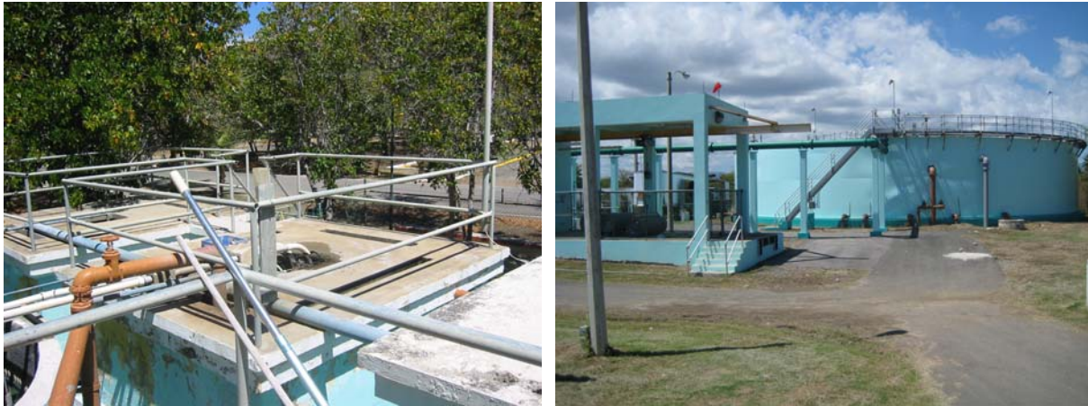
Figure 10. Small 3000 gpd sewage treatment plant at Cana Gorda Beach (left), one 750,000 gallon treatment tank within Guánica waste water treatment plant.
