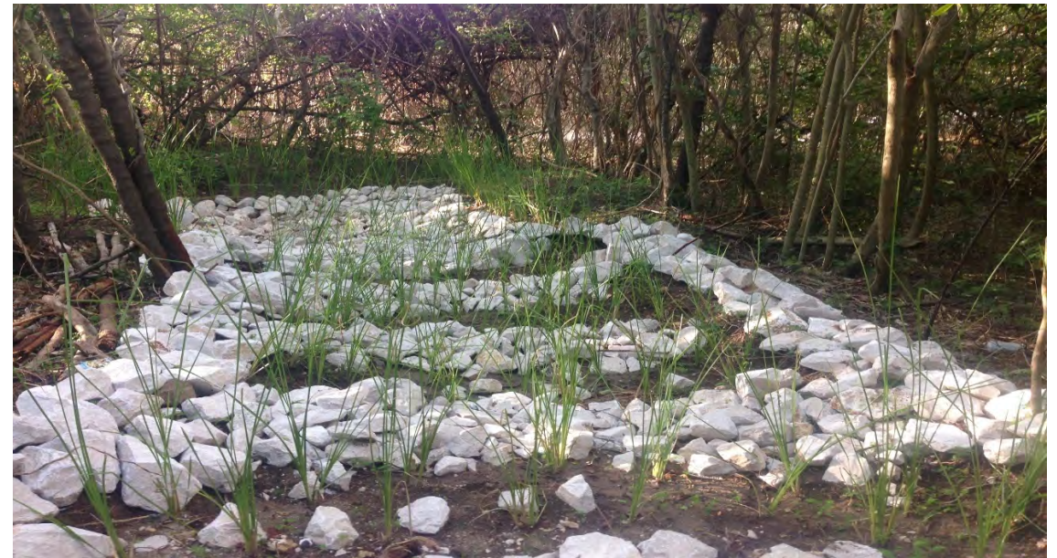
Figure 8. Vetiver outlet (rip rap aids to reduce flow velocities as do the vetiver plants as they mature) (Vetiver outlet for the Mosquito Bay Project in Vieques)
