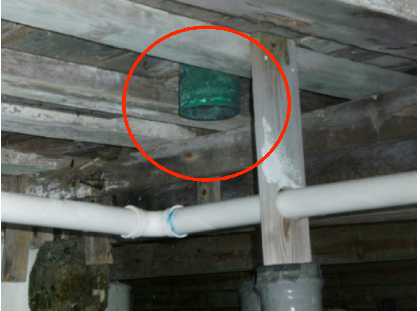
FIGURE 7: Suspicious open drainage. This is a possible pathway to any kind of household contamination including sewage and detergents.
