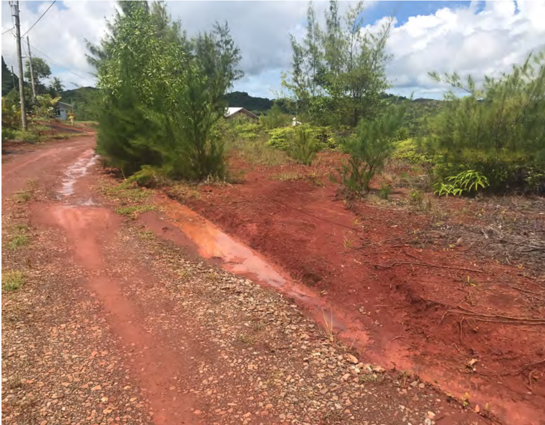
Figure 3. Location for rolling dip and sediment trap to reduce runoff volume and sediment transport on new development roads in Babeldaob (below is the restoration concept)
