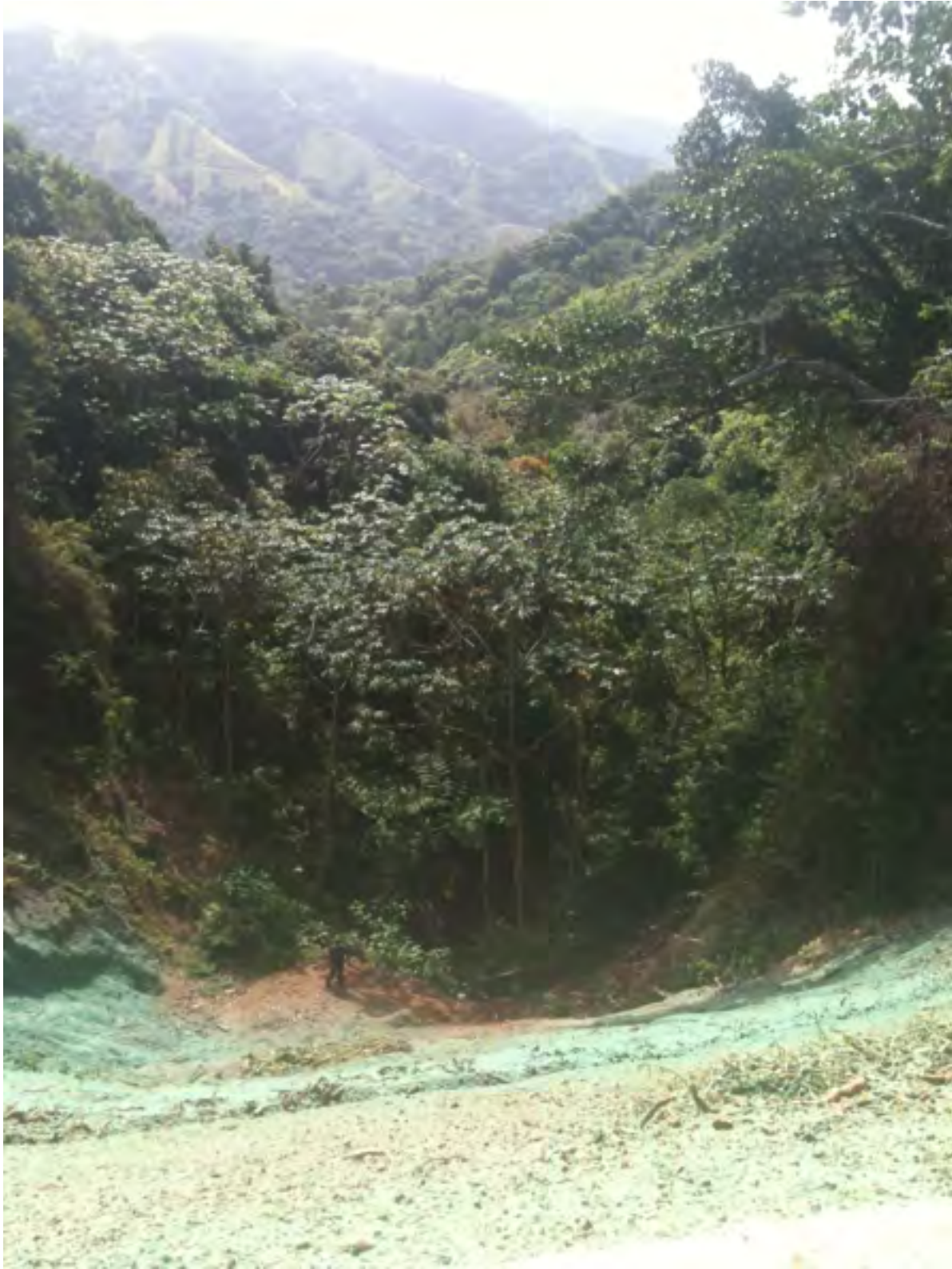
Figure 4. Hydromulching complete on the 70% slope plots
