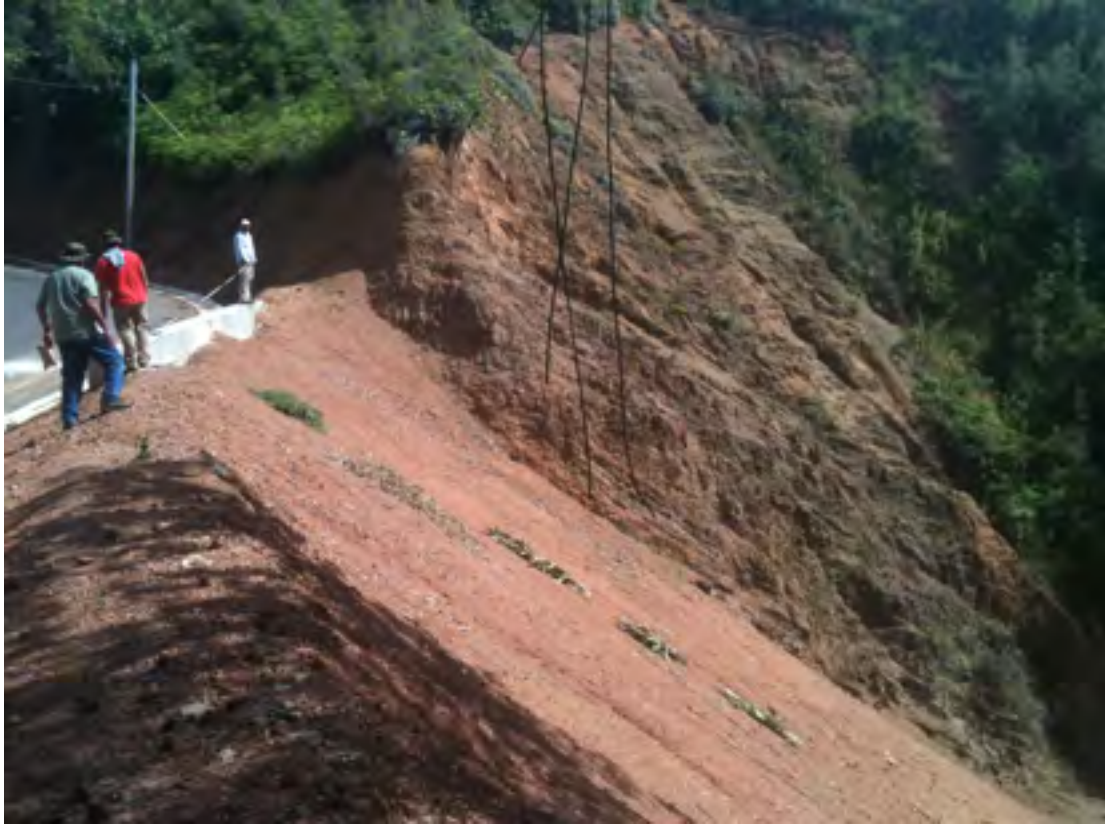
Figure 1. Laying out test plots on a 70-75% slope
