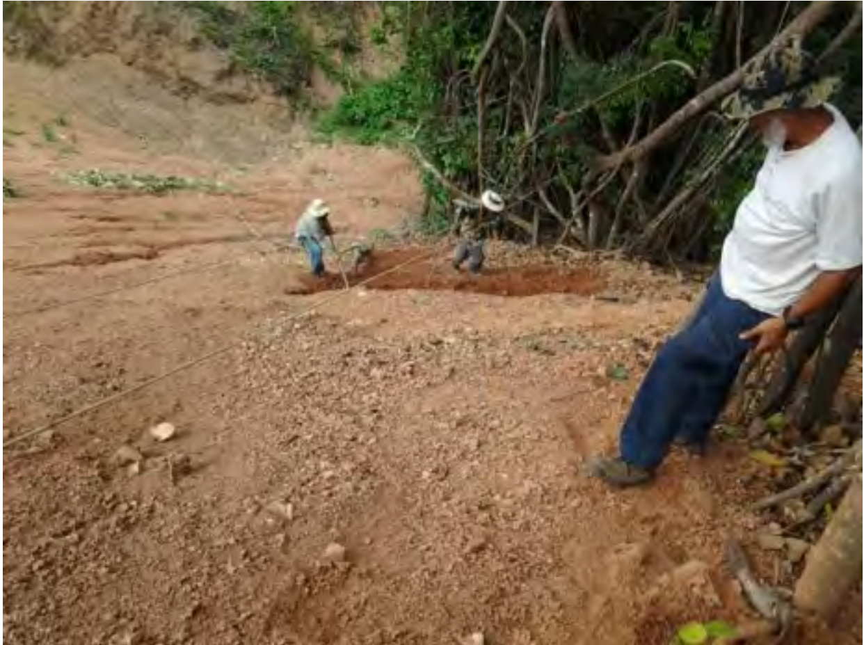
Figure 2. Breaking the slope to reduce concentrated runoff on the hillslope
