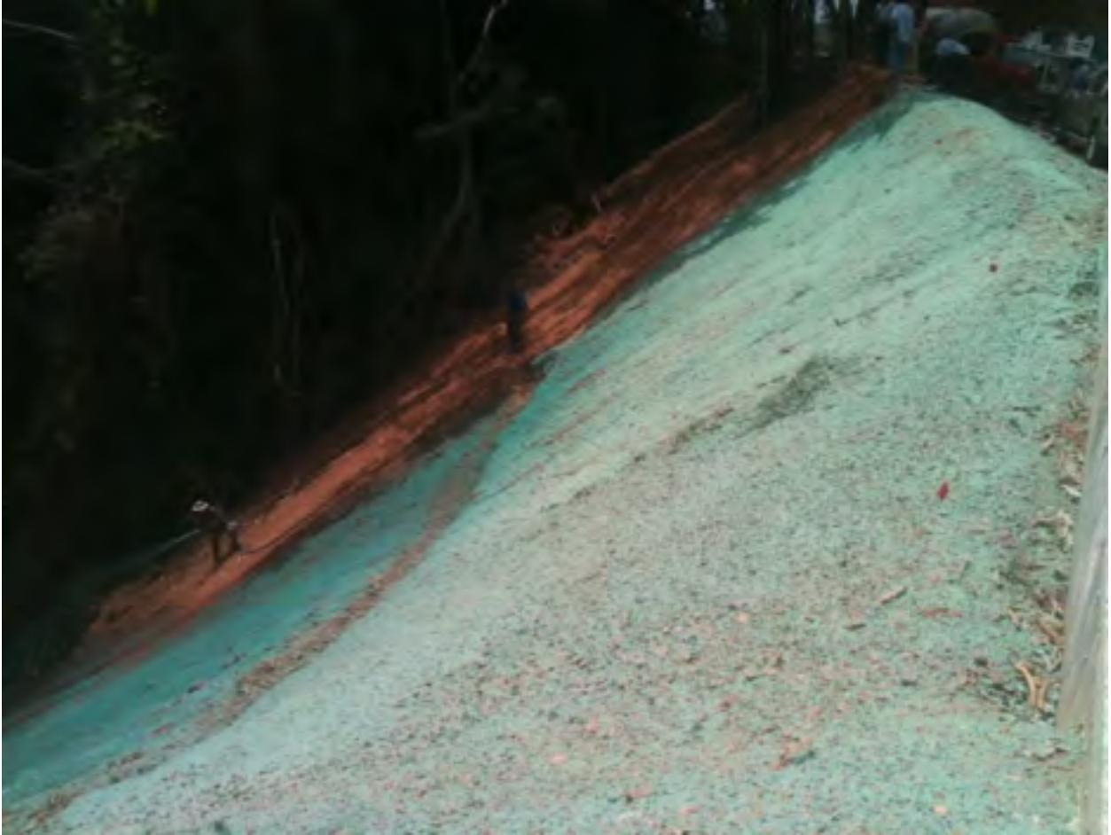
Figure 3. Flexterra application in the foreground and thick application of wood hydromulch in the distant plot (note red flags that delineate plots)
