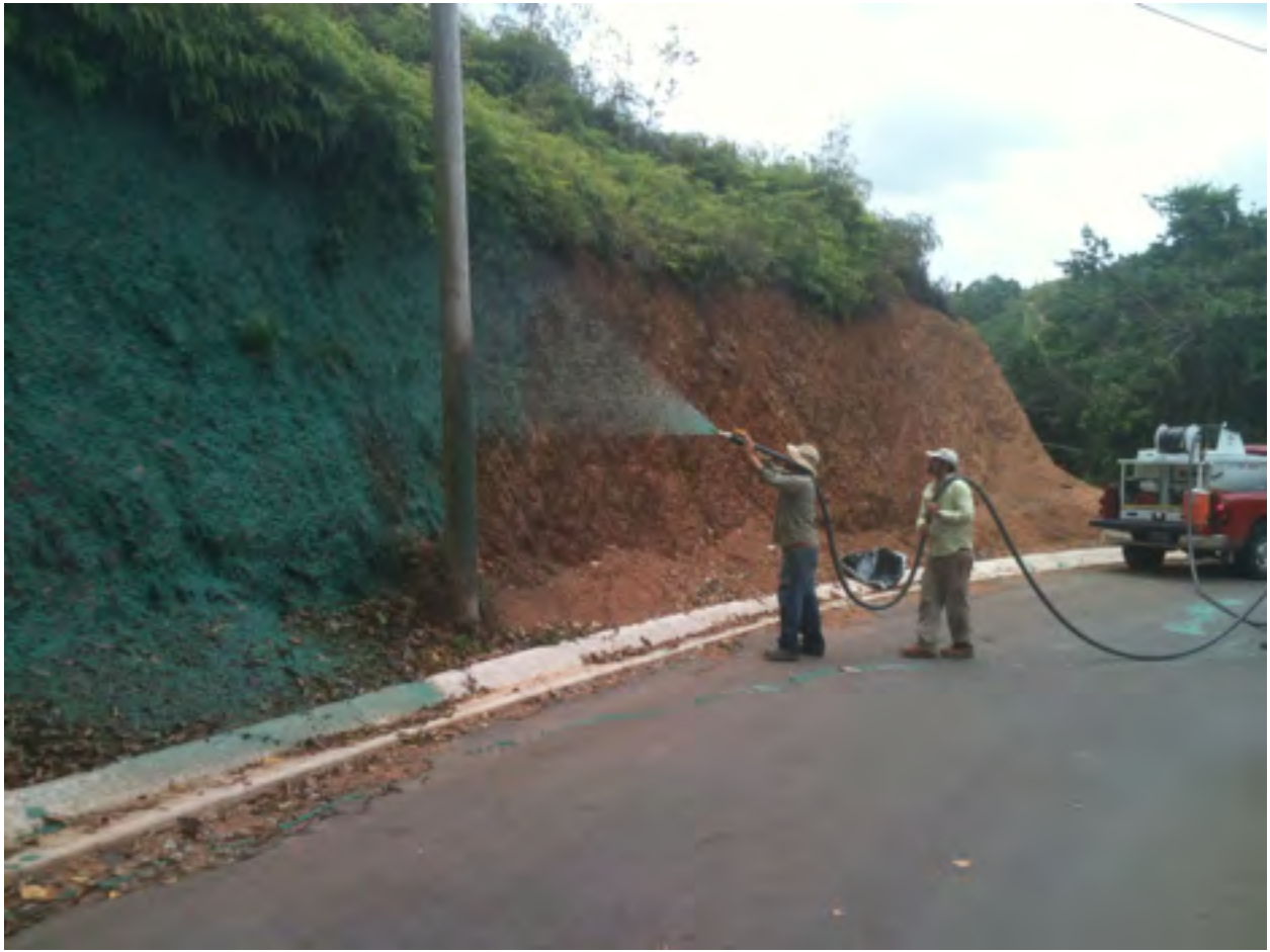
Figure 5. Applying hydromulch to the 85% slope in Plot #2
